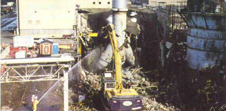
D.H. Griffin of Texas working on Utah sulphuric acid plant.
