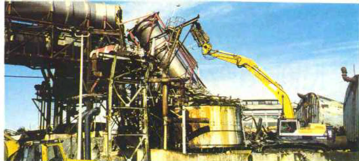
D.H. Griffin of Texas topples sulphuric acid plant.
