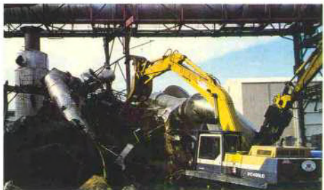
Using a grapple to clean the sulphuric acid plant
